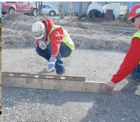
Step 5: Entire foundation must be flat and level. This critical step is best achieved with a laser level to ensure accuracy.
