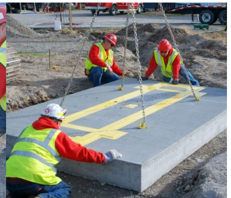
Step 6: Set 30m of builder's string line parallel to the approaches and install the scale along this line.
