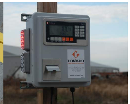
Step 9: Install controller on a suitable post, pole or wall and complete electrical connections. Apply power and weigh your trucks.
