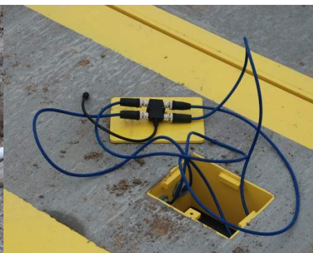
Step 8: Install home run cable from controller to 4 way connection. Terminate the watertight loadcell connections at scale and controller using the M12 screw on connectors.
